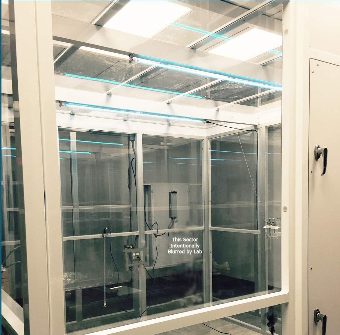
Two UVVC-L-160D 60" bulbs mounted on the ceiling of the NPAC
